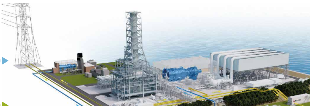
Takasago Hydrogen Park, Japan: A unique facility for hydrogen gas turbine R&D
