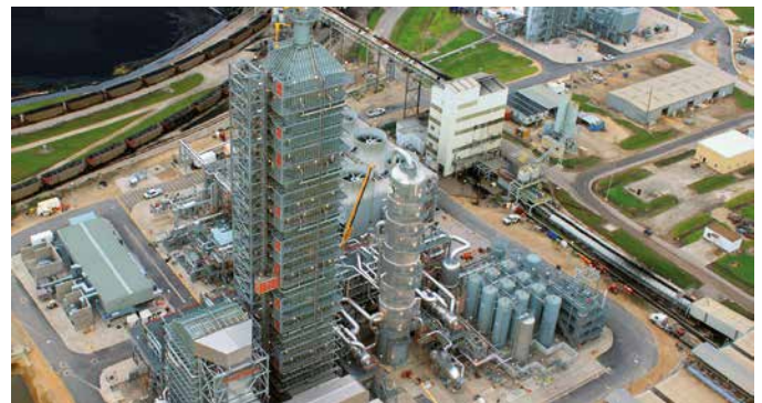
The world's largest CO 2 capture plant (Petra Nova/USA) with 4760 tpd capture
